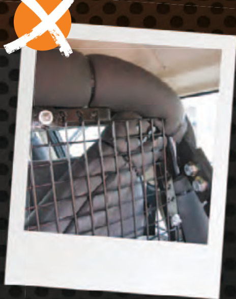
INSERT 21: Non rated mesh and non conforming brace coupler.
