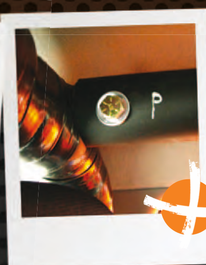
INSERT 9: Example of connection that is not fit for purpose and impedes head space.
