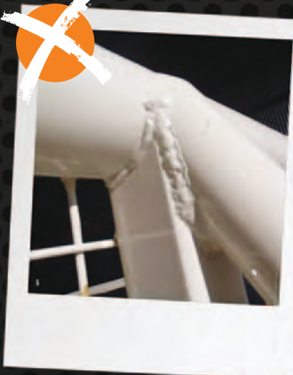
INSERT 22: Black pipe with non approved welding and non rated mesh.
