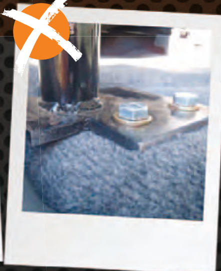
INSERT 20: Foot plate bolted over carpet with dangerous sharp edges.
