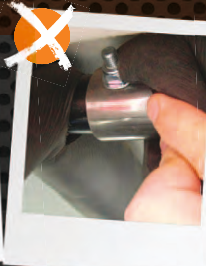
INSERT 8: Single bolt, through exhaust tube with airconditioning insulation as padding.
